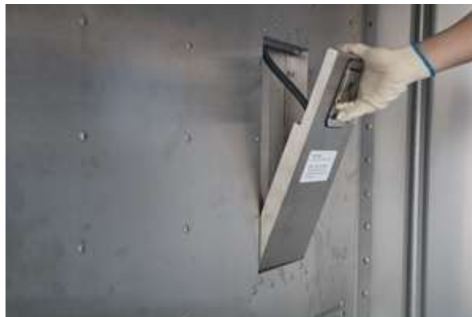
Figure 2.11.2. Mount Condensate Water Box
